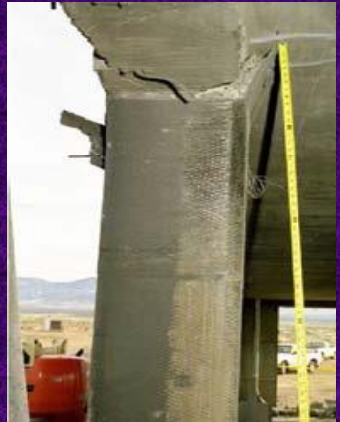
COLUMN WITH FIBRE WRAP
